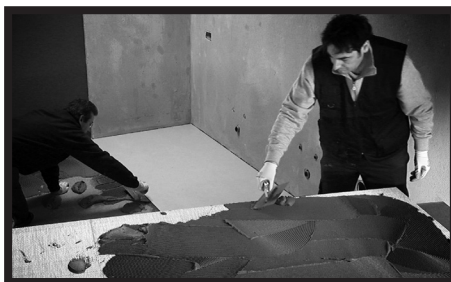
Fig.67 - Applying mortar to tile back
