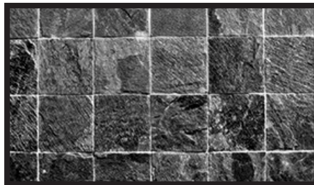
Fig.41/42 - Make sure that the substrate is sound and firmly fixed. Eliminate any residues of oil, grease or wax by washing with a solution of water and caustic soda followed by thorough rinsing. If chemical cleaning is not possible, adopt mechanical abrasion techniques.
