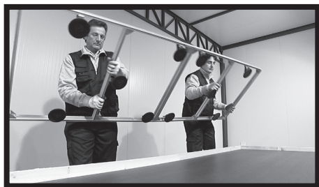
Fig.4/5 - All versions of THINNER gauged porcelain tile, of size 300x100 cm, can be handled by two people, using a special frame. Fix the frame to the gauged porcelain tile when it is still on the pallet using the suction cups. Raise the frame and gauged porcelain tile to eliminate the suction effect.
