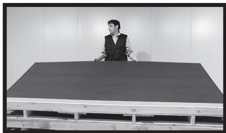
Fig.1 - All types of 300x100 cm THINNER gauged porcelain tile can be lifted by one person. Lift the gauged porcelain tile with open hands. Slowly raise the longer side so as to eliminate the suction effect, due to contact with the underlying gauged porcelain tile, and ensure a good grip.
