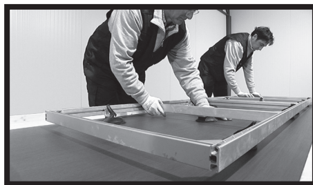
Fig.4/5 - All versions of THINNER gauged porcelain tile, of size 300x100 cm, can be handled by two people, using a special frame. Fix the frame to the gauged porcelain tile when it is still on the pallet using the suction cups. Raise the frame and gauged porcelain tile to eliminate the suction effect.
