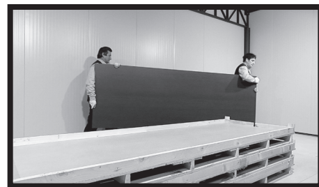
Fig.3 - When the slab is upright, hold it from its top edge and shift it keeping it straight and upright. This operation should be performed with the aid of a second person.
