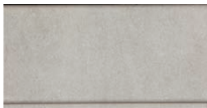
2381 I Concrete Cove Base & Corner
