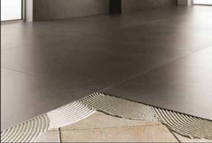
Install Over Existing Floor Tile
