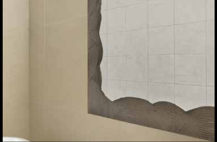
Install Over Existing Wall Tile
