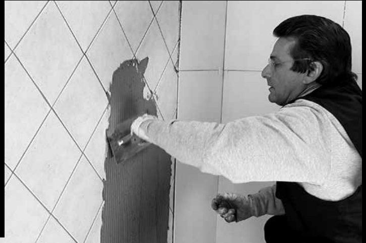
Install Over Existing Wall Tile
