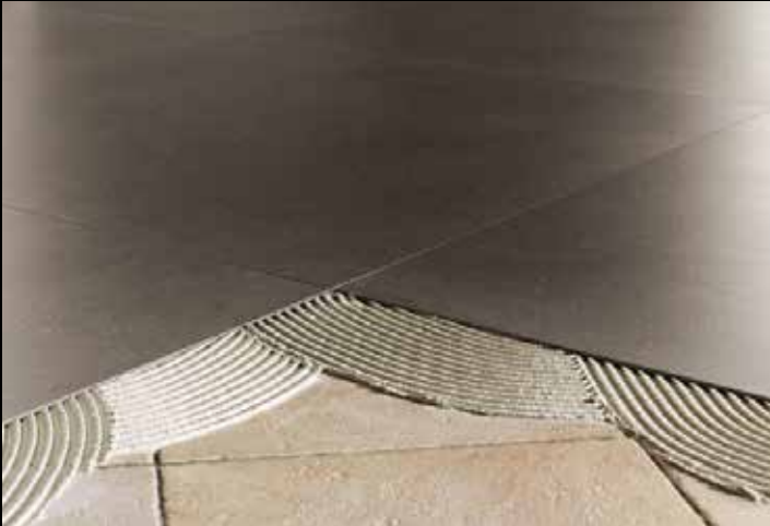
Install Over Existing Floor Tile
